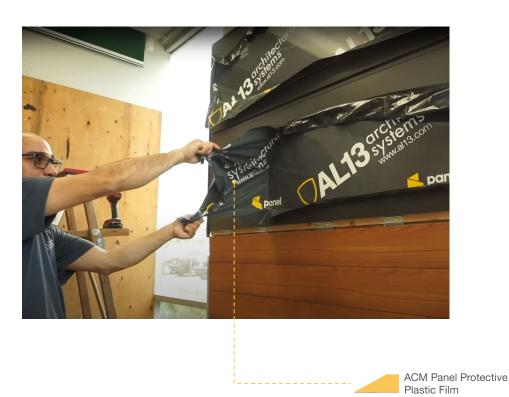
Once the install is complete, work from the top down to remove the protective plastic film and clean the panels as required. Take note of any installation flaws and ensure all top caps are fully hammered into place.
