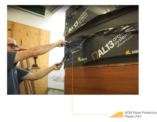
Once the install is complete, work from the top down to remove the protective plastic film and clean the panels as required. Take note of any installation flaws and ensure all top caps are fully hammered into place. Protective film must be removed once install is complete.
